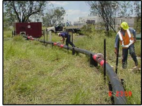
BHP, BMA coal processing plant supplied by the dam water and the Hydrosmart system installed next to the dam on its 200mm pipe work.
