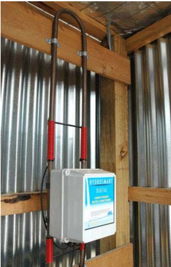
A 20mm Hydrosmart installed on the Moore's property at Strathfieldsaye, near Bendigo, showing the free flow through the unit.
