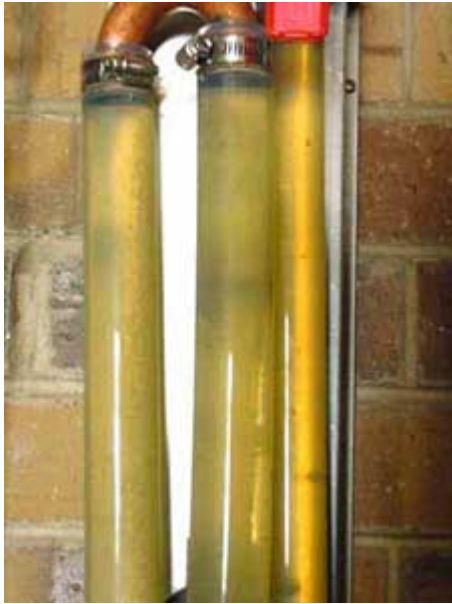
UV system with scale and bio-film build up.
