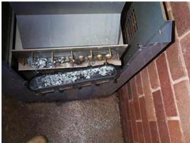
Scale in cover shown before installation Dec 2009
